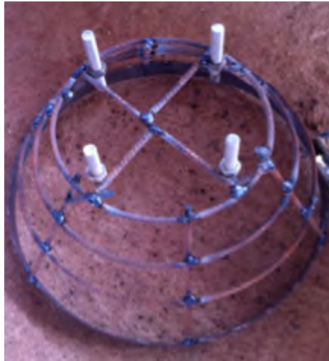
Figure 35: Finished metal cage
