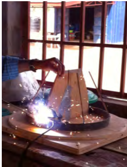
Figure 31: Welding steel rod to the base ring
