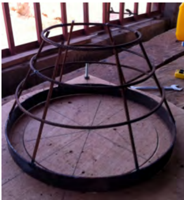
Figure 33: Metal cage, not yet finished
