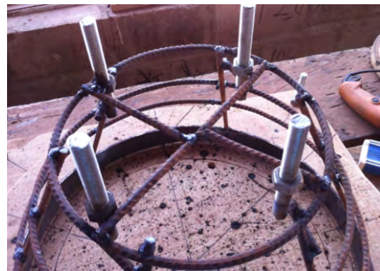
Figure 34: Metal cage, with threaded rods
