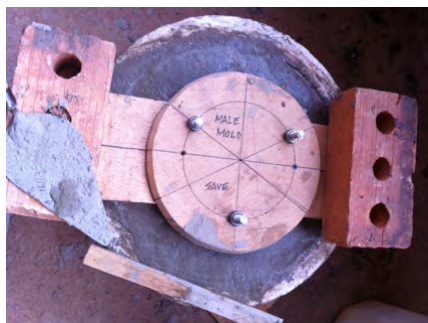
Figure 47: After pouring concrete into the cavity
