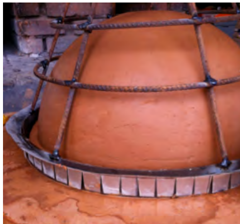
Figure 39: Metal cage over prototype; Item C around base of steel ring
