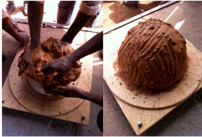
Figure 36: Preparing and applying clay onto the Item A
